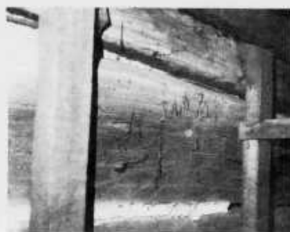
Interior view of original oak logs, still sound, in the attic of the Bergquist cabin
